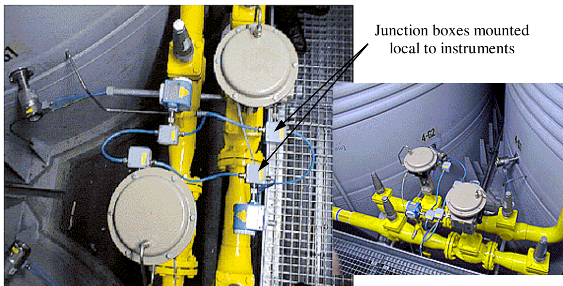
Typical PA Installation using junction boxes
